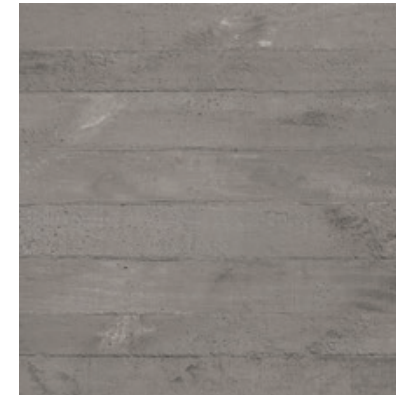
FORMWORK | COFRADO - PK16903RT [R12C]
