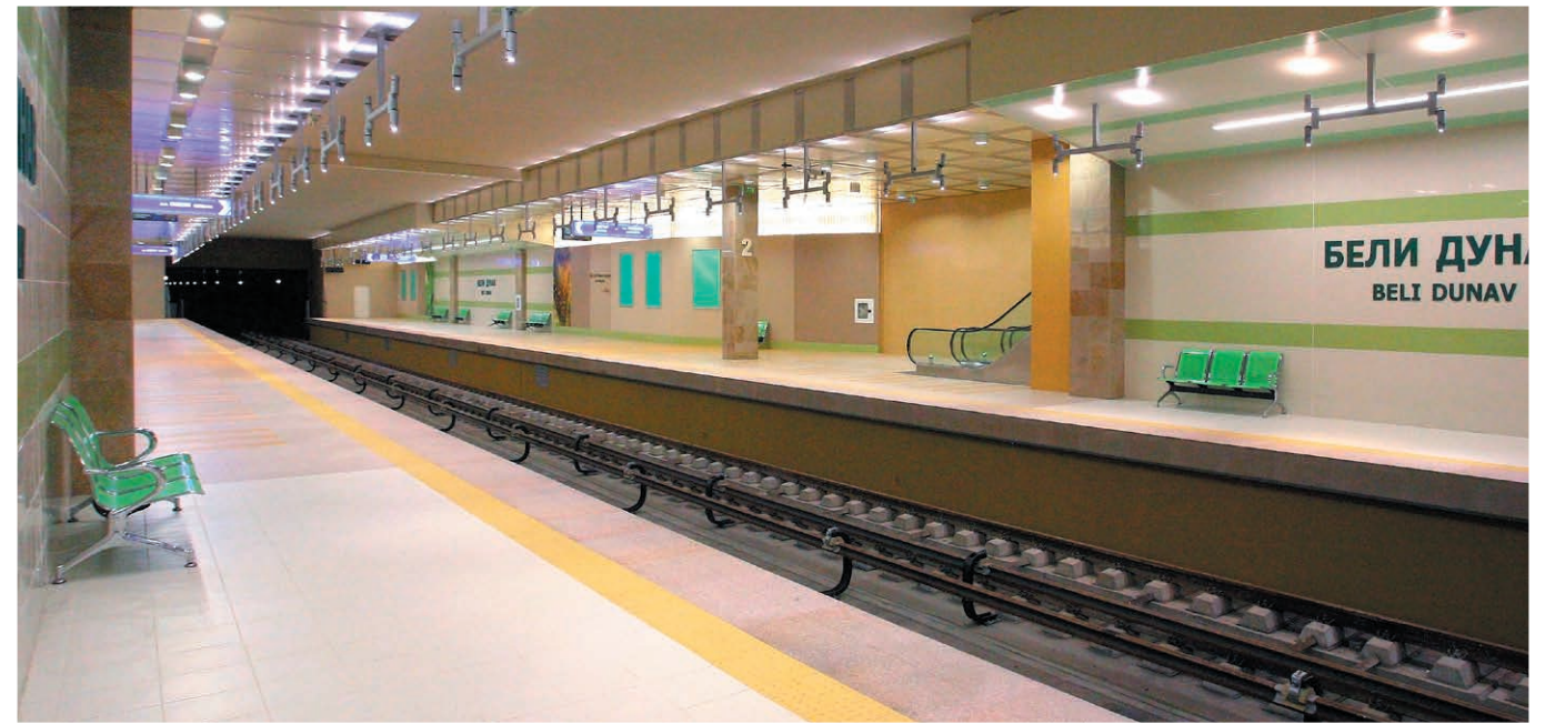
BELI DUNAV METRO STATION Sofia, Bulgaria
