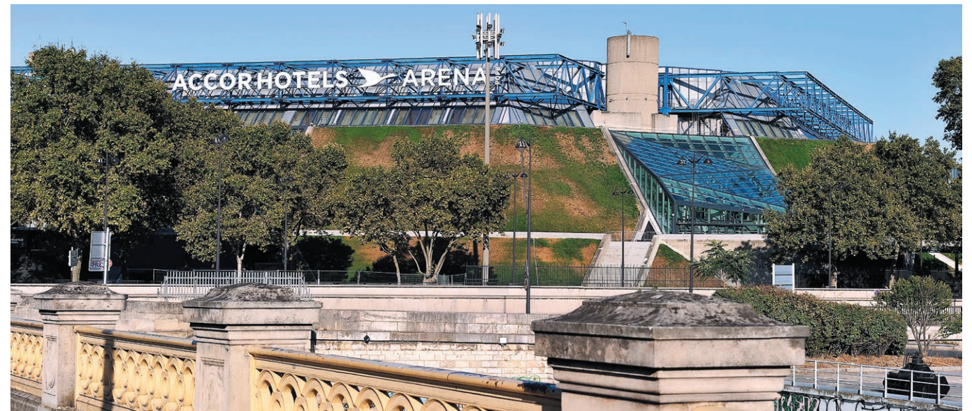
ACCOR HOTEL ARENA BERCY Paris, France
